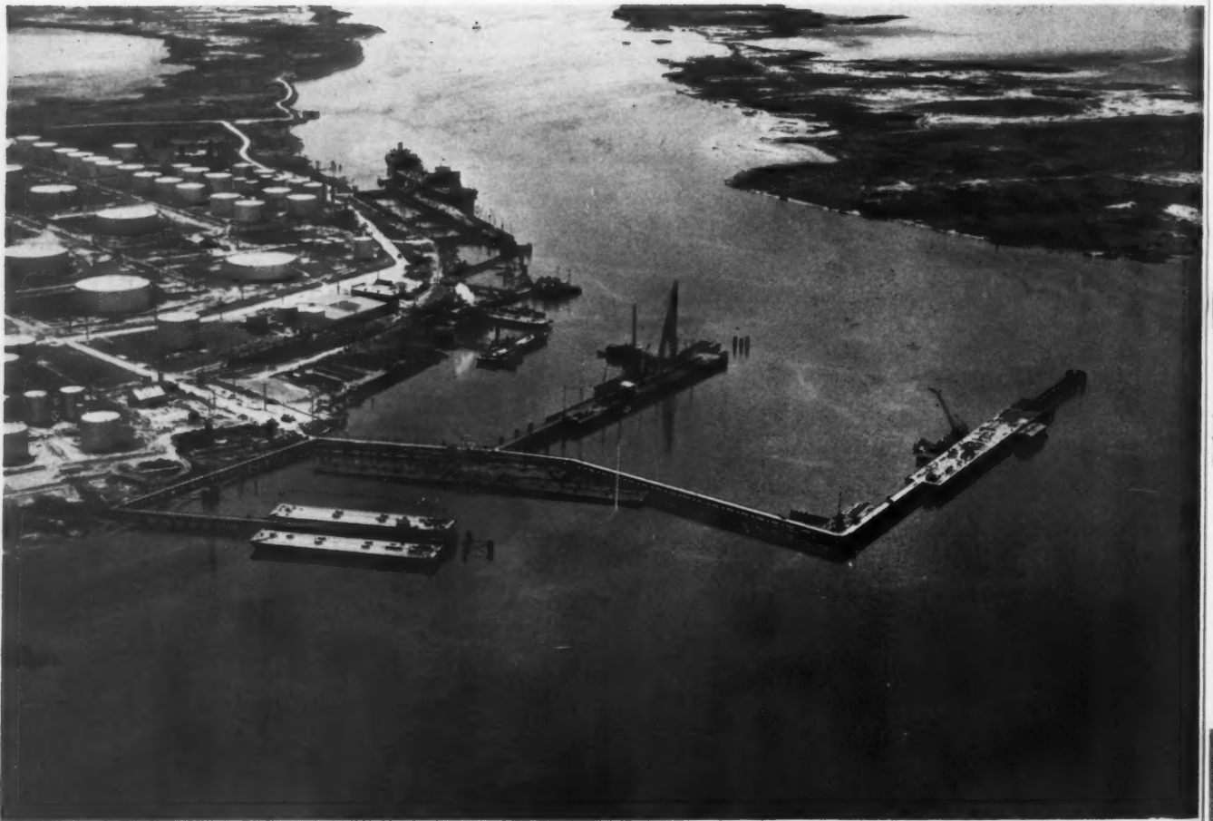
NEW DOCK at right, built at Baytown for the Crude Oil Department, will be big enough to accommodate two of the largest tankers now afloat and even bigger tankers planned or under construction. From this new dock in Houston ship channel will go still more oil to the nation's markets.
